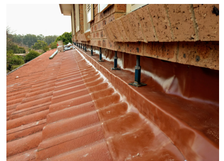
Figure 14: Straight Flashing Reinstallation
