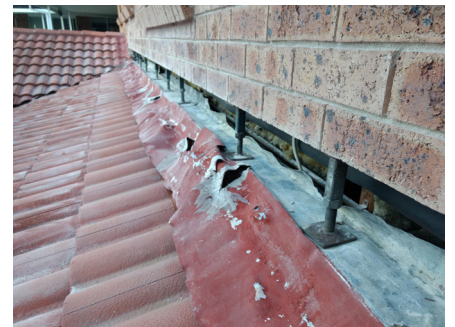
Figure 13: Straight Flashing Damaged Due To Poor Installation
