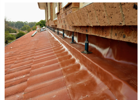
Figure 14: Straight Flashing Reinstallation
