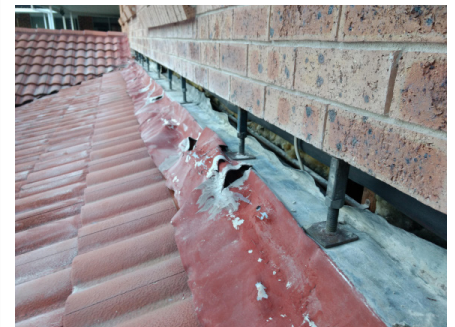
Figure 13: Straight Flashing Damaged Due To Poor Installation
