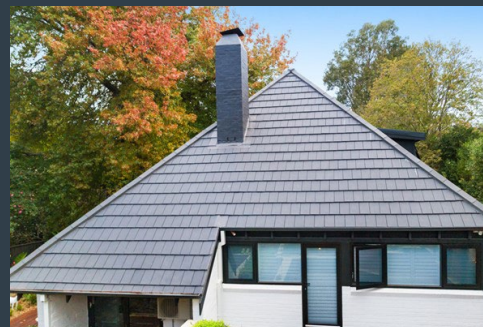
Light Coloured Concrete/Terracotta Roofing Tiles
